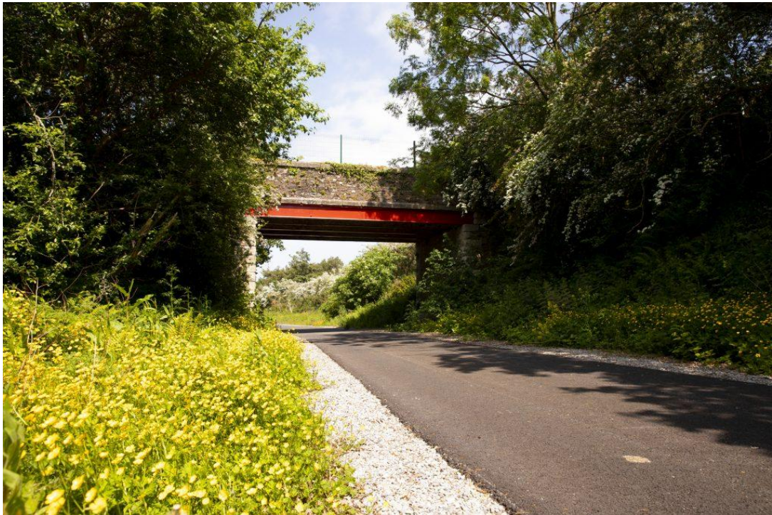
Figure 4-17 - Finished Pavement and Edge Treatment; South East Greenway, County Kilkenny / County Wexford (Source – South East Greenway [Visitors Homepage - South East Greenway])
