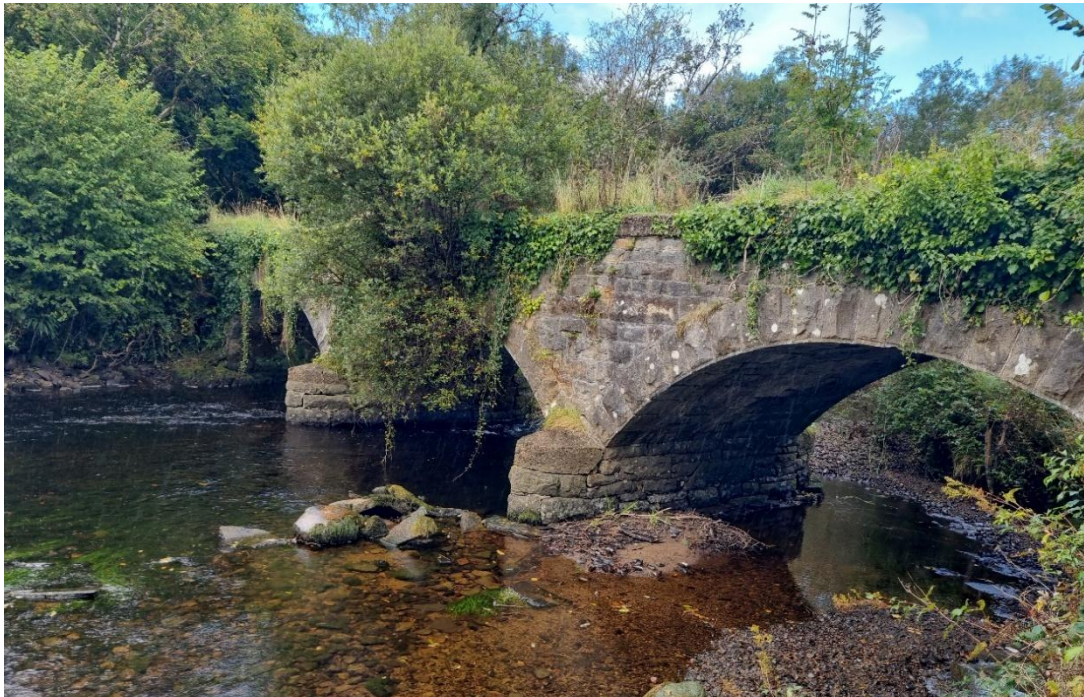
Figure 4-2 - Existing Railway Bridge Structure at River Eske in Donegal Town (S01)
