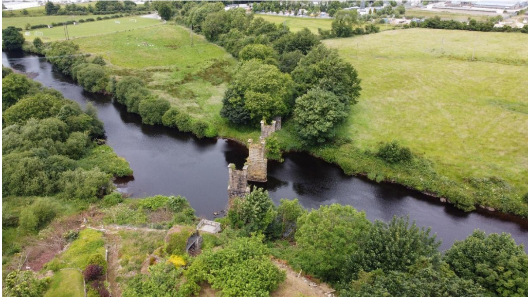
Figure 4-8 - Existing Railway Piers in River Finn (S20)
