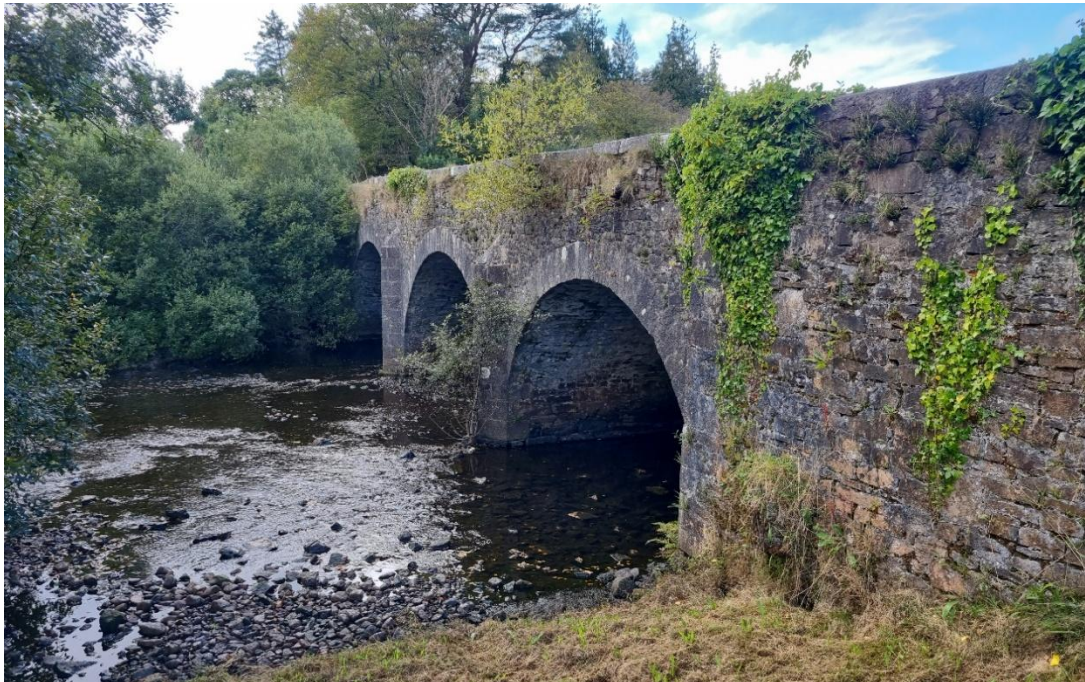
Figure 4-4 - Existing Road Bridge over River Eske (S05)
