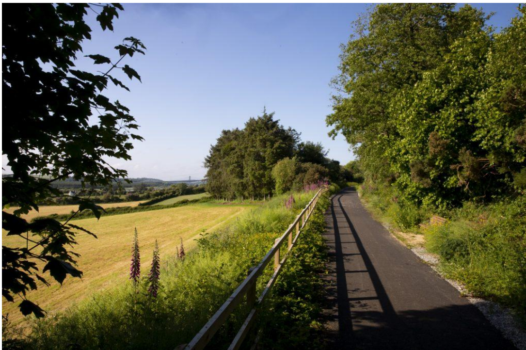
Figure 4-18 - Finished Pavement; South East Greenway, County Kilkenny / County Wexford (Source – South East Greenway [Visitors Homepage - South East Greenway])
